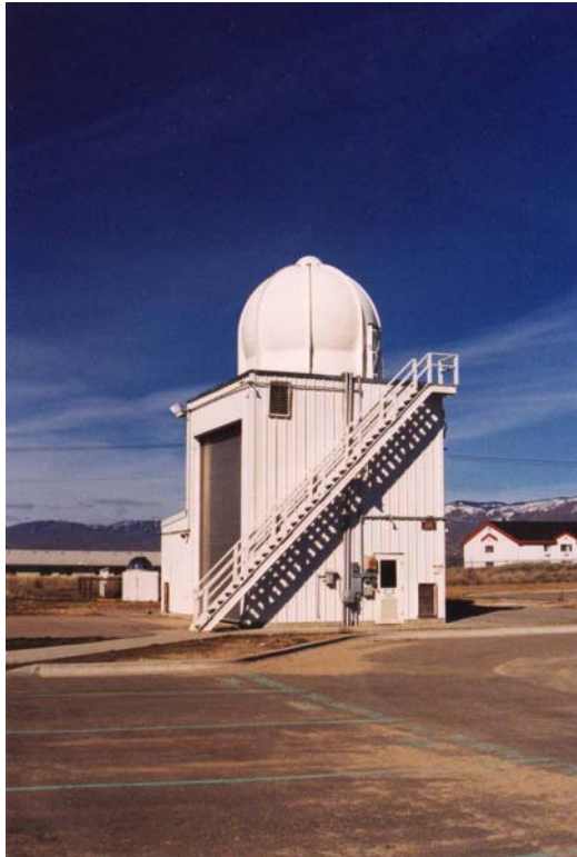
A radome (radar dome) - a weatherproof enclosure used to protect an antenna.
